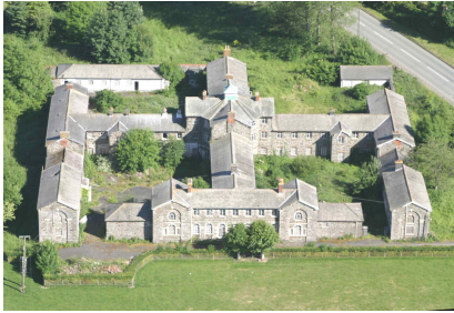
The Lanfyllin Union Workhouse, which was one of our Top Ten Endangered Buildings for 2007 and has since received a grant
