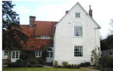
Manor Farm, South Stoke: West Elevation
