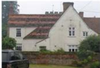
Manor Farm, South Stoke: North Elevation.
