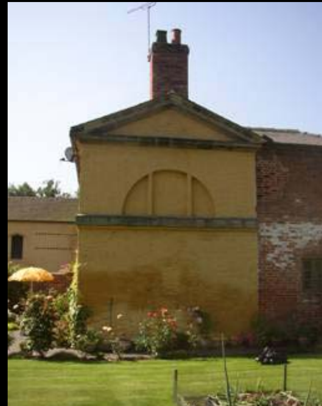
There is no evidence of any timber frame surviving within the west elevation. There is a very faint indication that the tie beam and collar of the roof truss have been retained within the masonry.
