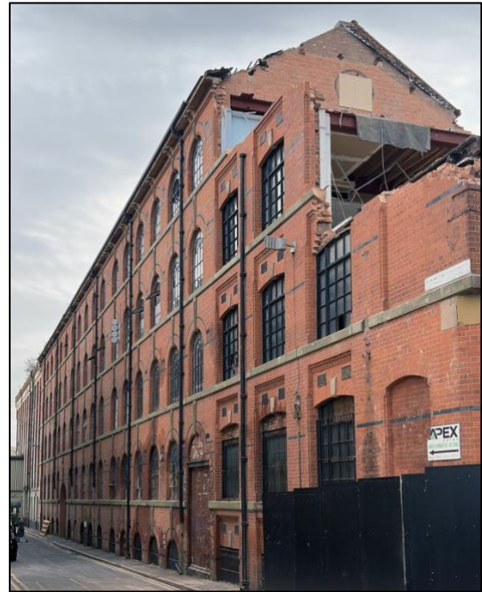
Figure 2: The original building on Wheat Street with the damaged building in the foreground (photo: Colin Hyde).
