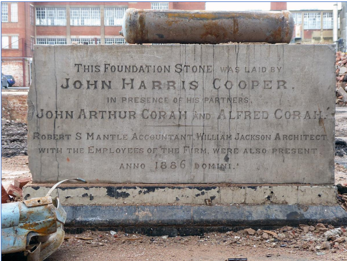
This 1886 foundation stone was left after the debris had been cleared. Photo: Colin Hyde.
